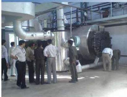
3-PASS FULLY WET BACK
