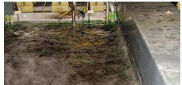
Eductor Agitation showing lack of foam and clean surfaces
