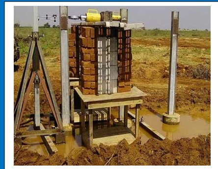
Pile Load testing Arrangements at Construction Site
