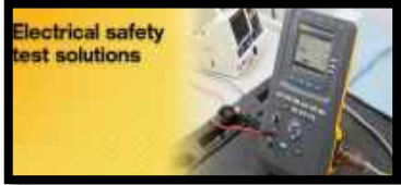
Electrical Safety Audit
