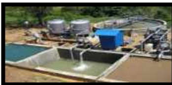
ETP Integrity Inspection
