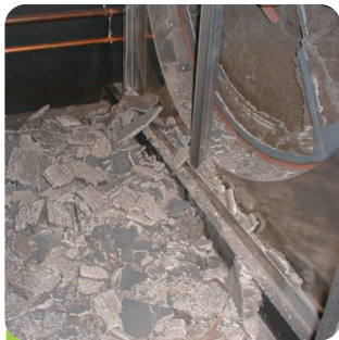
Step 1 Removal of old cores of desiccant
