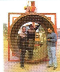
Fabrication and Drilling
