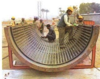
Adhesive application and fixing
