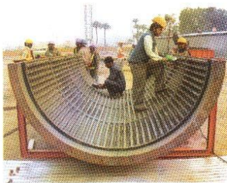
Adhesive application and fixing
