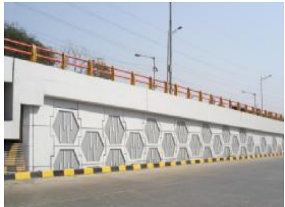
Reinforced Earth wall
