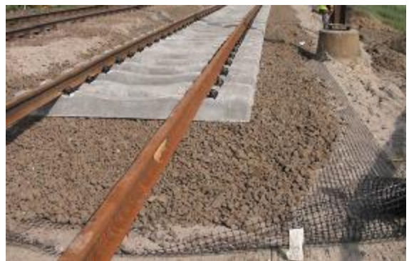
Base reinforcement for railway tracks
