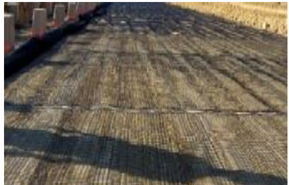
Base reinforcement for paved roads
