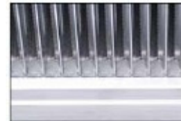
Completely joint sealing
