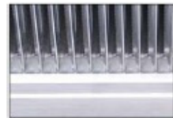
Completely joint sealing
