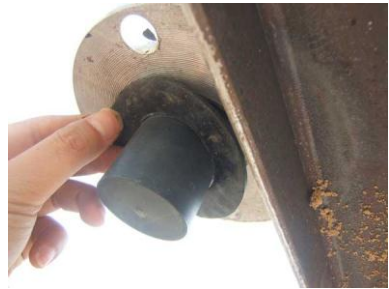
⑧ Finished installation of transducer
