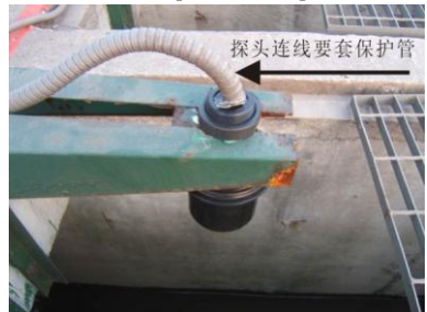
② the connected the probe with protection tube
