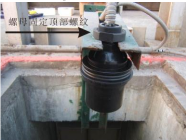
① fix the top thread with the nut
