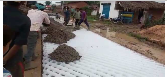
Filling Concrecells with RMC equipment
