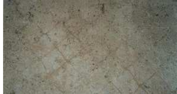
Finished Surface with Concrecell
