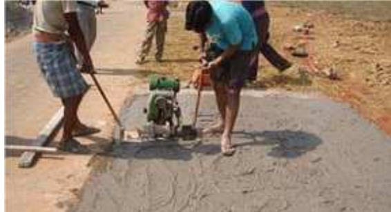
Vibrate Concrete with plate vibrator
