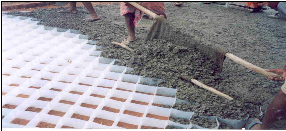
Fill M-30 Concrete into Concrecells
